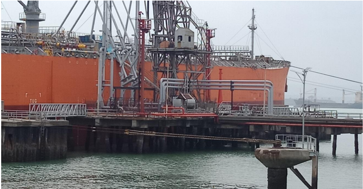
An oiler being decanted at Mombasa Port Oil Jetty. It takes about 4 days to offload an oiler carrying 50, 000 tons of fuel.
