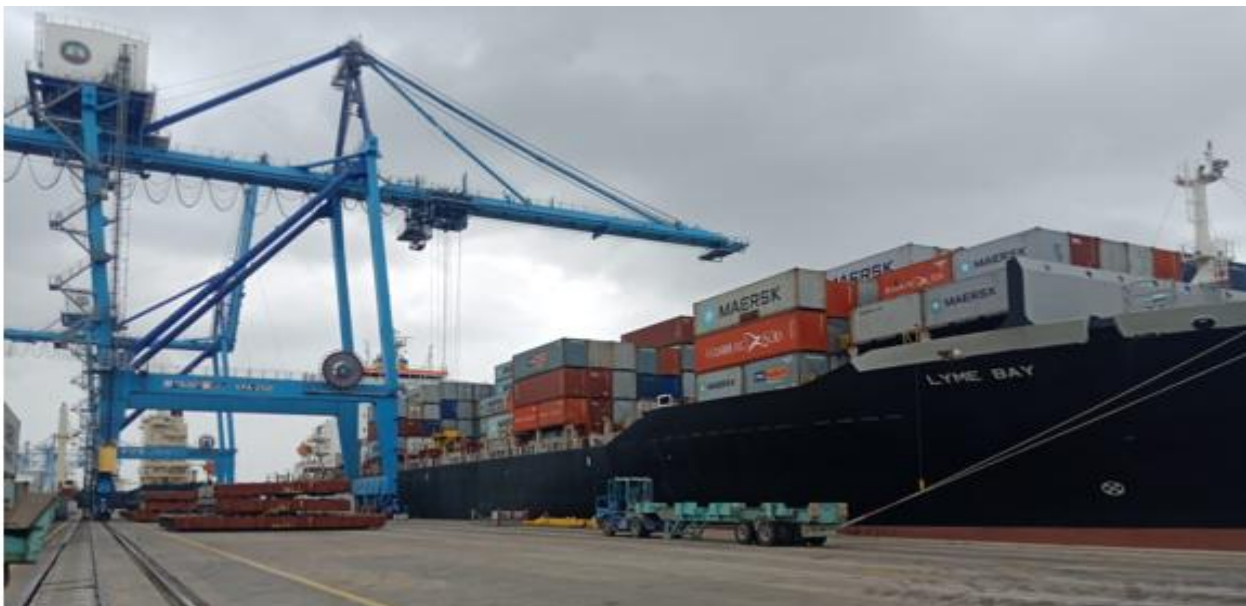
A vessel being served at the new container terminal at Mombasa Port. Following dredging of the Port and construction of a bigger berth. The Mombasa Port can now receive Post Panamax container ships of capacity 8,000 TEU's
