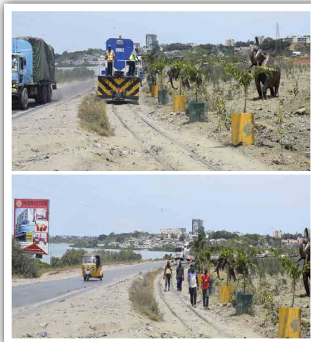
Figure 7: Absence of a barrier between the road and railway line posing a safety hazard to pedestrians.
