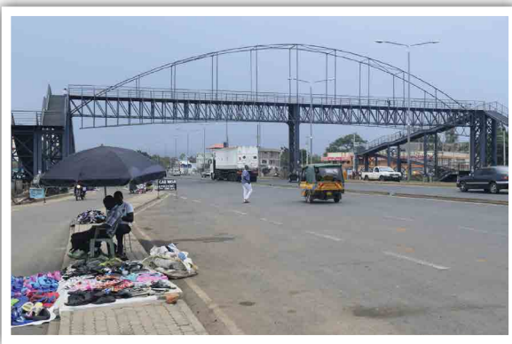
Figure 33: Pedestrian dangerously crossing the highway at grade despite provision of a footbridge
