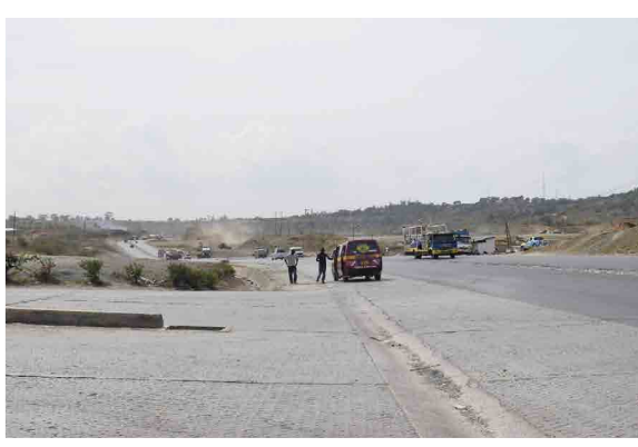
Figure 10: Picking up/dropping off of passengers at non-designated locations (no provision for a bus bay)
