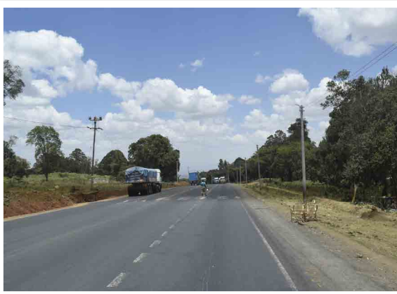
Figure 26: Hawkers/vendors selling their products on the carriageway around Sachangwan area oblivious of the safety hazards
