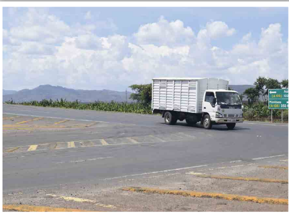
Figure 15: Lorry exiting towards Oloitoktok from the A8 Highway (note the skid marks indicating difficulties when making the turn)
