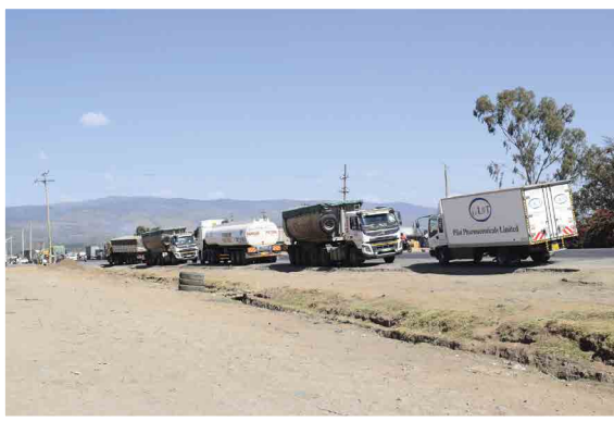
Figure 25: Heavy trucks parked on the shoulders effectively narrowing the carriageway and impairing visibility for other road users
