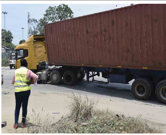
Figure 4: Insufficient turning radius for heavy trucks at Makande Junction
