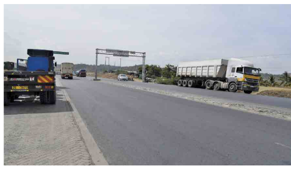
Figure 8: Faded road markings
