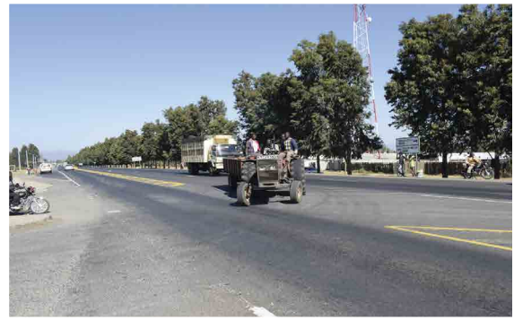
Figure 24: Lack of a provision for an accelerating lane for Eldoret bound traffic from Njoro
