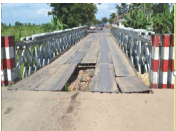
Left: March 2013 , the single lane bridge without pedestrian walkway at Gatumba/Kavimvira border station at the Burundi-DRC border crossing point was in need of repair, NCTTCA survey team had recommended upgrade to increase its capacity.
