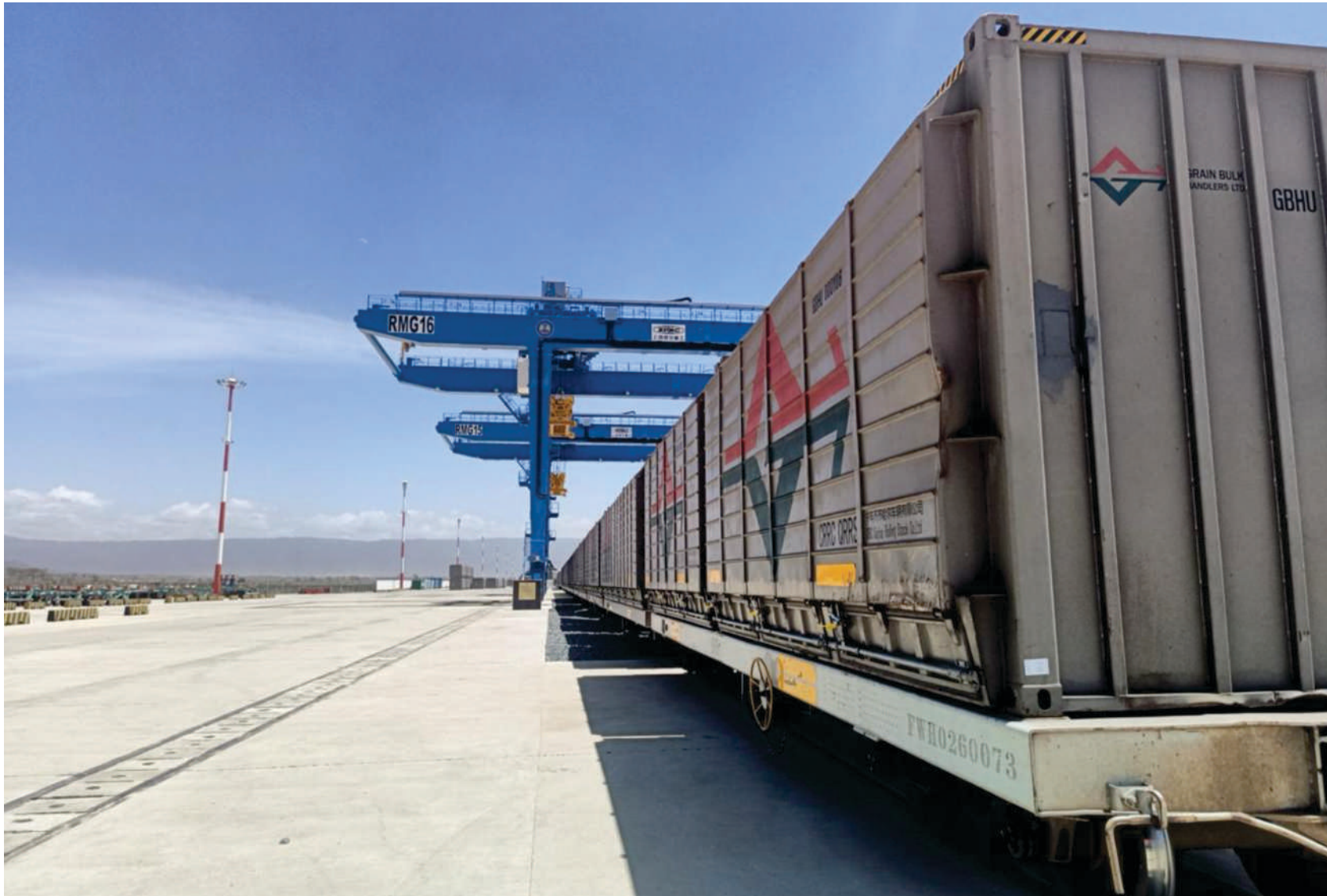
The Naivasha Inland Container Depot (ICD), commissioned in 2020 and linked to the Port of Mombasa via SGR/MGR rail lines, serves as a key transit node for Uganda, Rwanda, South Sudan, and DRC. It boosts cargo throughput by over 2 million tonnes annually and eases Mombasa port congestion.
