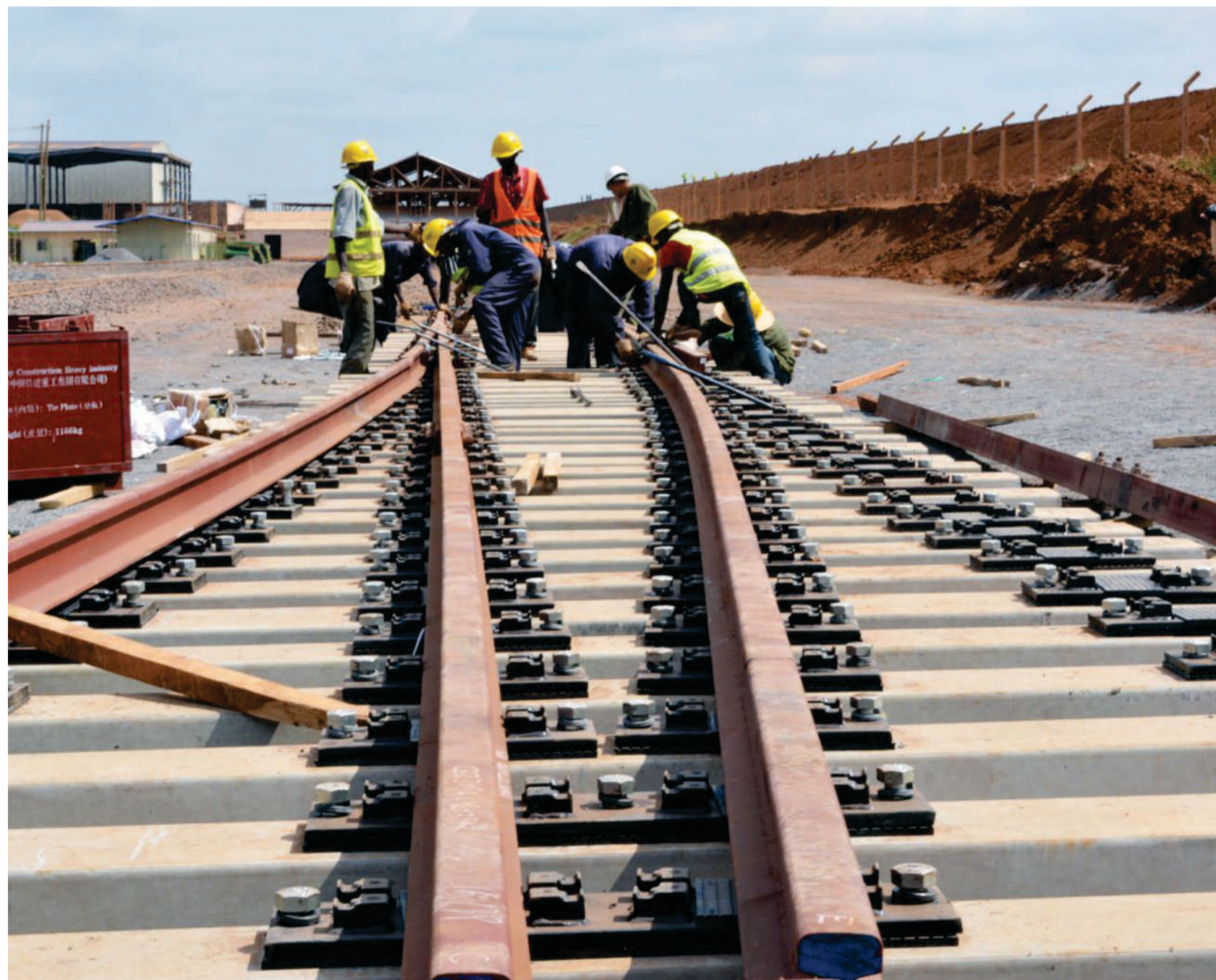
Workers captured busy with the construction work on a Standard Gauge Railway (SGR) line, installing rails onto concrete sleepers to progress the East African SGR Rail Network.
